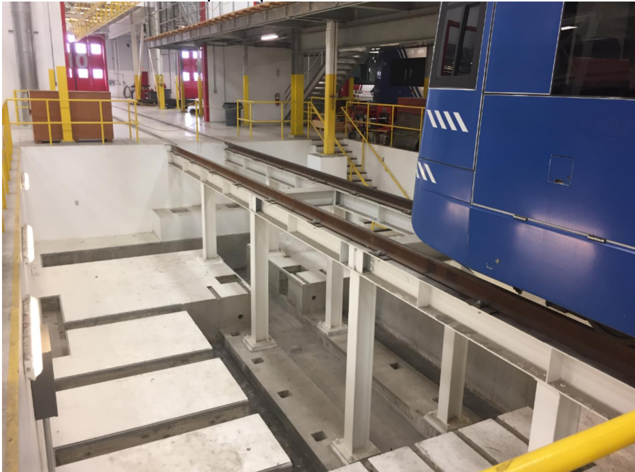
Photo inside of UTA's rail car repair shop – note the clean white floors
